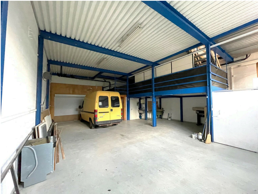
rez - mezzanine visible
